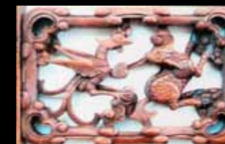
Fig. 6 Detail of the openwork of nineteenth-century wooden window frame from Jiangxi Province. (Collection of Daniel C. K. Lau)
